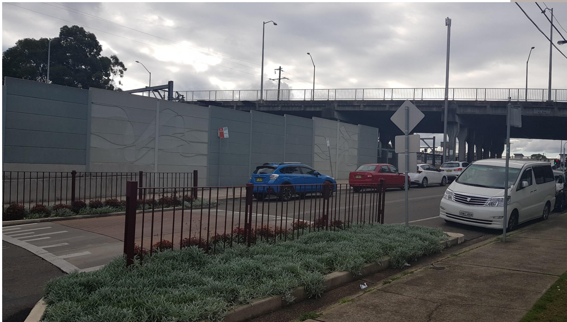
Figure 3 - Existing Hebel Sound Panel Around Railway Corridor
